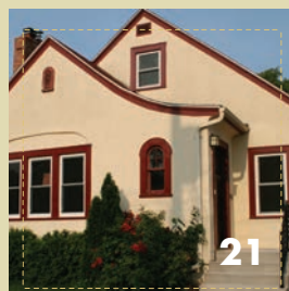
Heritage Homes Restoring Neighborhoods One Home at a Time
